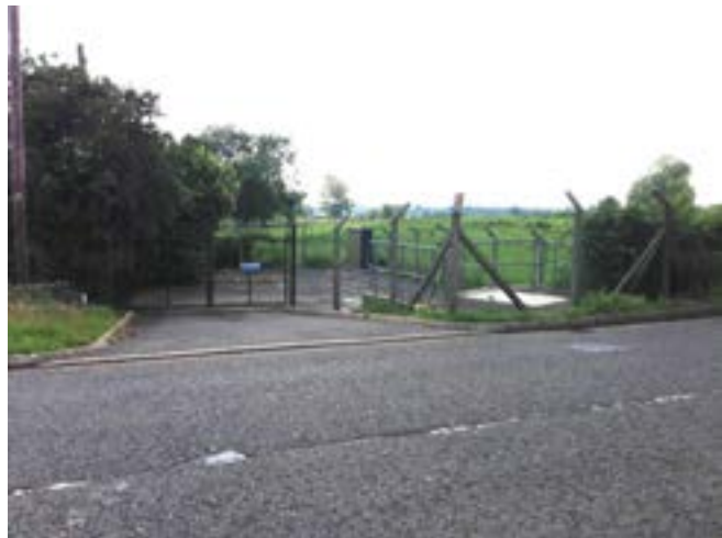
Pumping station located adjacent to the site off Station Road.
