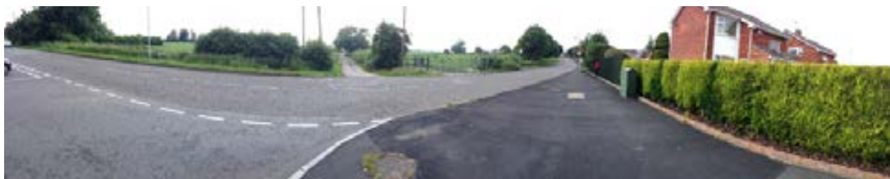
The site is a backdrop to views from Thorndale opposite.
