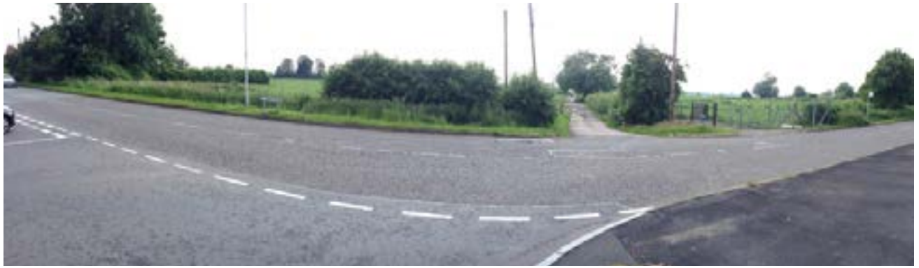
Existing farm access and pumping station on Station Road.
