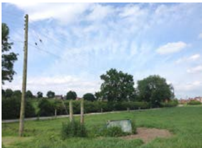
Overhead cables alongside the farm access track.
