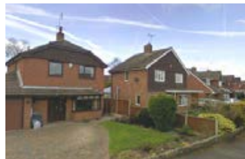
2 storey detached houses located on Gateway Avenue typifies architectural vernacular and palette of materials.
