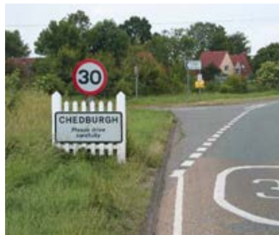
Example of fixed gateway upon approach into village with 'please drive carefully' signage.
