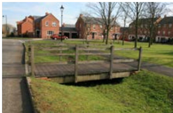
Swale, Sustainable Urban Drainage.
