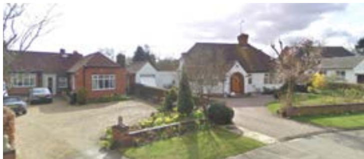
Bungalows located on Sandyfields. Elevational design and use of materials varies.
