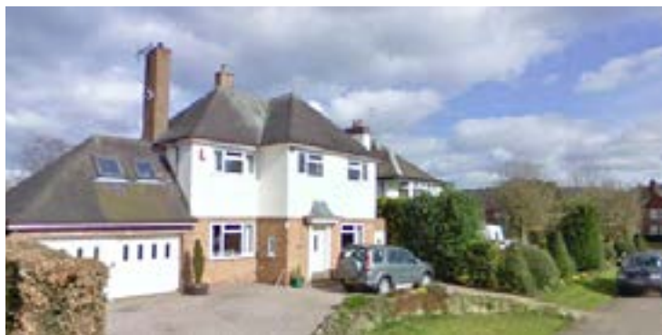
Large detached houses in Sandyfields set away from the streetscape. Building separation distances across the street are greater which in conjunction with frontage landscaping, which promotes a 'leafy feel' to the street.
