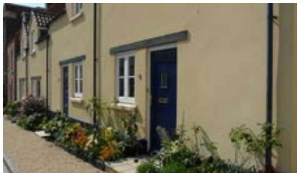
Dwellings close to pavements with narrow defensible planting.
