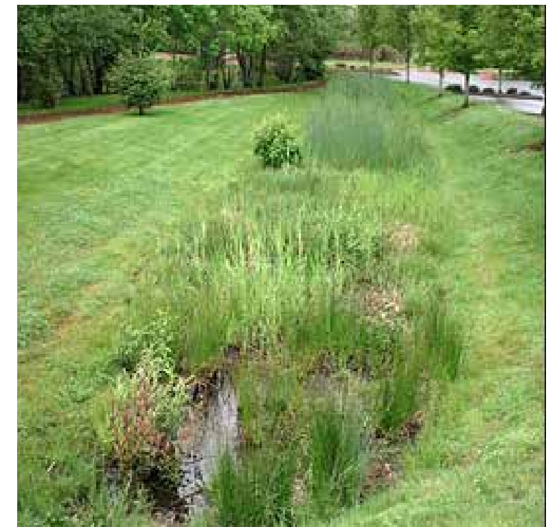
Example of a detention basin with micro ponds
